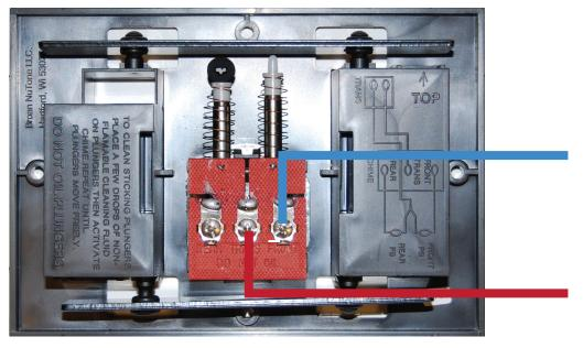
Wire from SkyBell attaches to terminal marked "Front Door".
